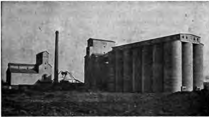
A modern elevator.
